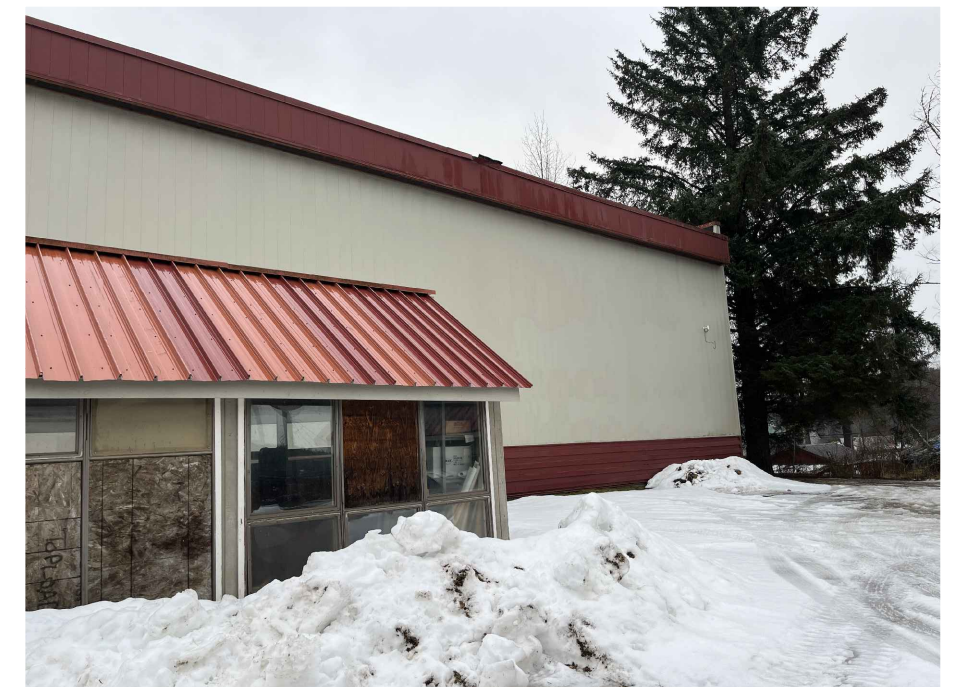
PHOTO 6: WEST WALL, VIEW LOOKING EAST
