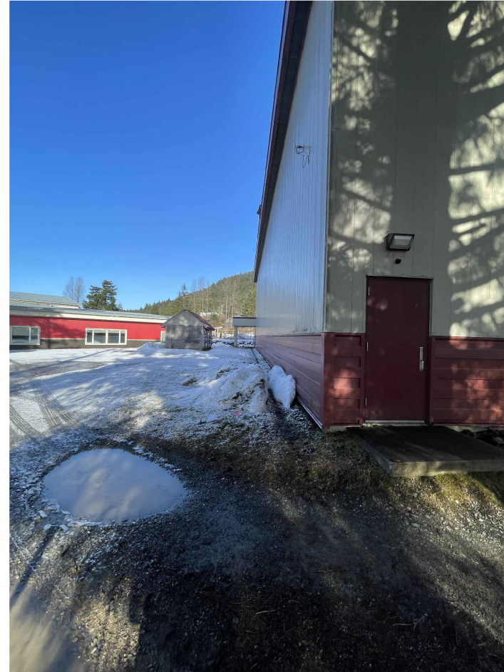
PHOTO 3: WEST WALL & TRUCK HAUL AREA
