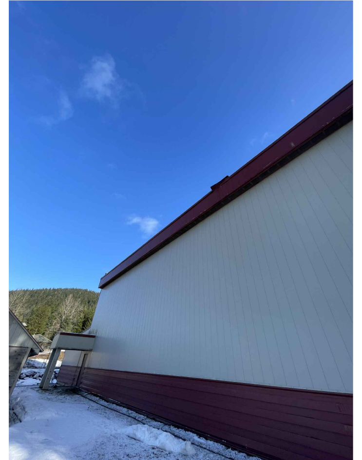
PHOTO 4: WEST WALL & TRUCK HAUL AREA
